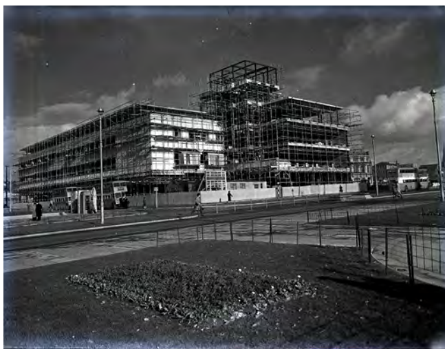
The steel frame in place for construction of Dingles, 1950 (Ref: 1418/06138 © Mirrorpix, The Box, Plymouth)
