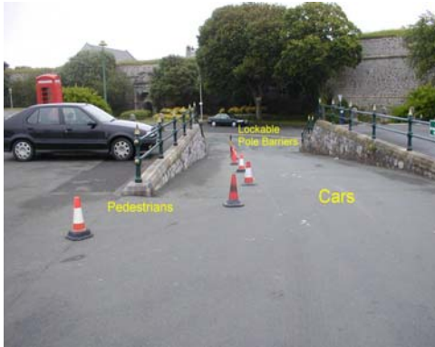
Photograph C- Overall viewpoint of Hazards
