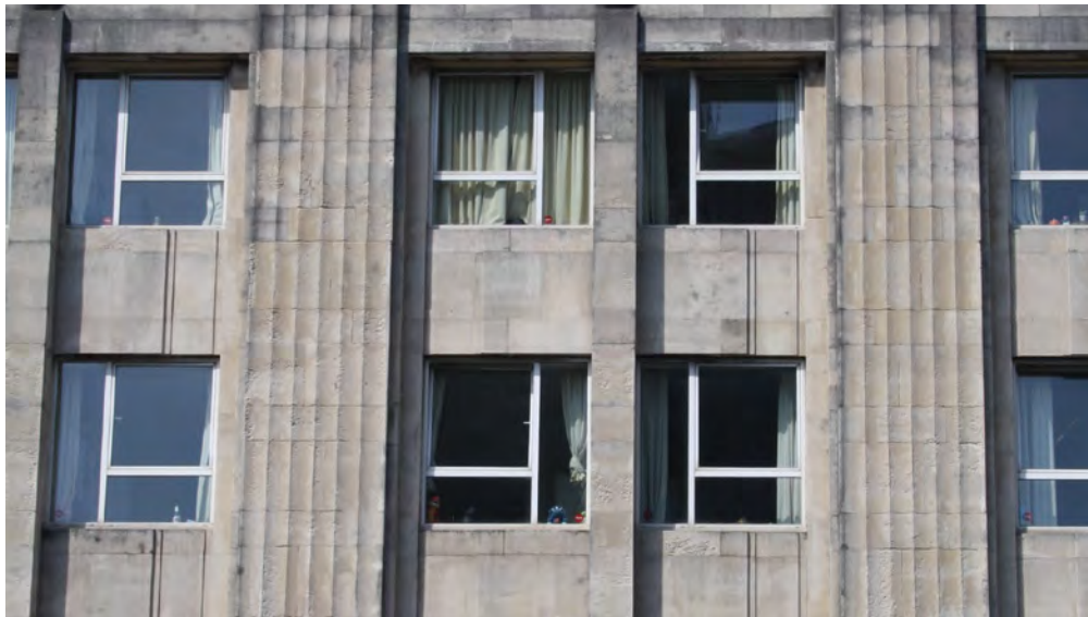
Pollution is causing staining to the Portland stone of buildings which line the street
