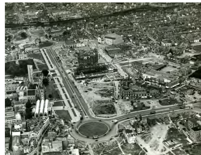
Aerial shot of Royal Parade, c.1950 with New George Street under construction. The steel frame of Dingles is in place. The old market is still standing. (Ref: 3488/7065 The Box, Plymouth)
